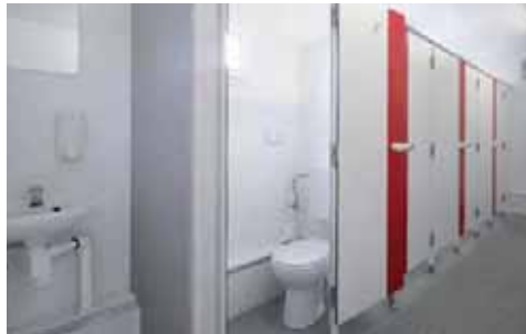
KITCHEN & SANITARY INSTALLATIONS
